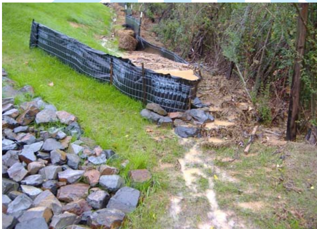
A silt fence J-hook is very effective in containing sediment and can save on installing greater lengths of fence.
