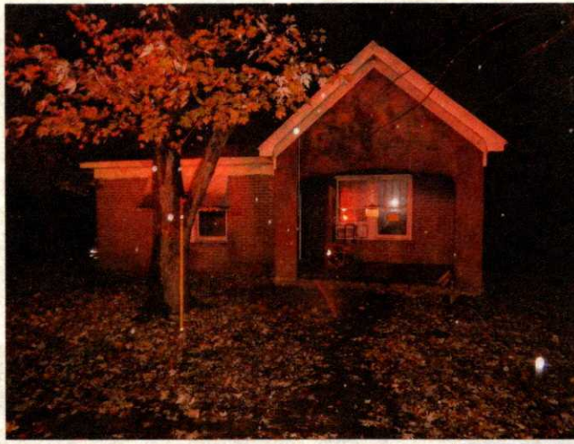
Left photo: Front of house fire on Pinewood 12/3/20
