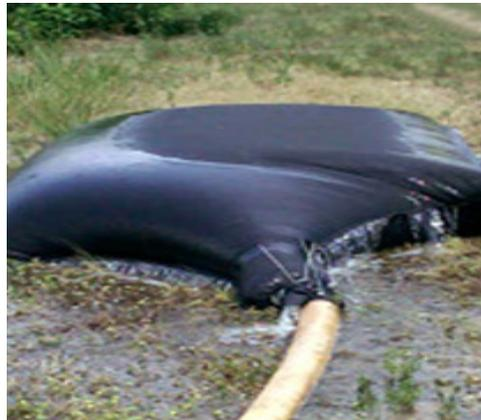
EPA, ADEQ, and The City of Hot Springs requires that all discharged water associated with dewatering activities must be processed through a filtering device before entering a storm sewer system. Filter bags, (as pictured above) gravel, fiber rolls, or grassy areas may be utilized to improve water quality.
